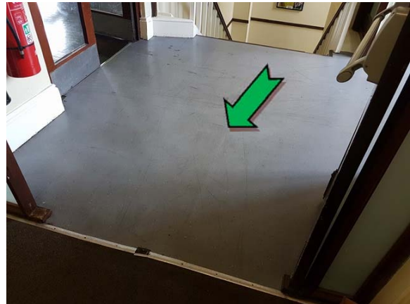
Photo 4. Interior, level one, south stairs, floor – assumed non asbestos-containing sheet vinyl.
