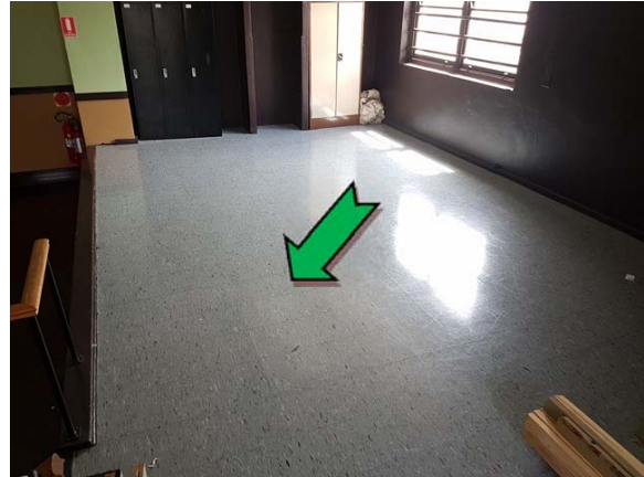
Photo 2. Interior, level one, hall, floor – non asbestos-containing vinyl floor tiles.
