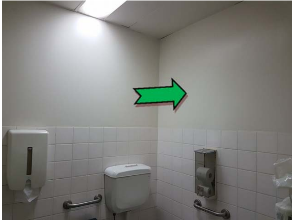
Photo 7. Interior, ground level, staff toilet, wall – non asbestos-containing fibre cement sheeting.
