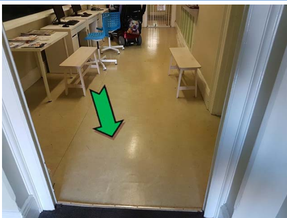
Photo 11. Interior, ground level, reception office, beige floor coverings – non asbestos-containing sheet vinyl.
