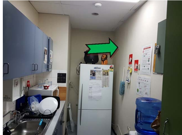
Photo 8. Interior, ground level, kitchen, wall – assumed non asbestos-containing fibre cement sheeting.
