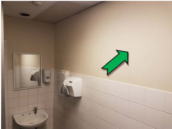
Photo 3. Interior, level one, toilet, walls – assumed non asbestos-containing fibre cement sheeting.
